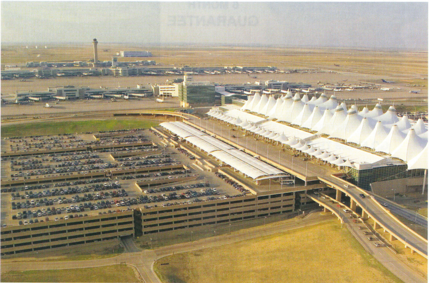
Three of DIA's six garages, all undergoing moisture-protection restoration to extend the lives of the structures.
