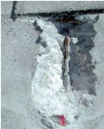
Fig. 7: Severed strand revealed after exploratory opening was made (magnetic scanning image of the same strand is shown in Fig. 5)
